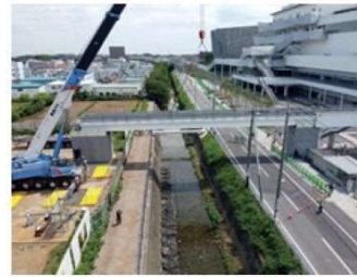
Long bridge construction
