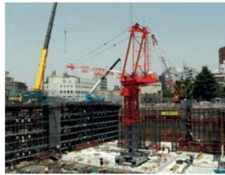
A scenery of construction
